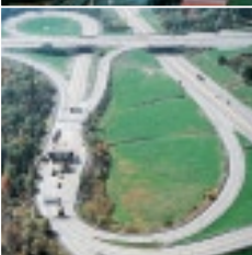
Pennsylvania Turnpike - Pennsylvania, USA
