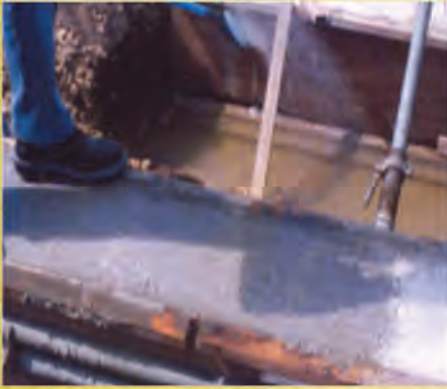
BRUSH OFF DIRT AND WET CONCRETE JOINT.
