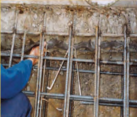
SLOWLY PRESS ON TO CONNECTING SLAB JOINT.
