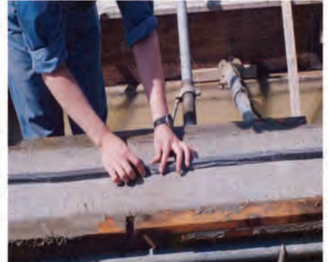
CONNECT TWO PIECES BY END-BUTT JOINING.
